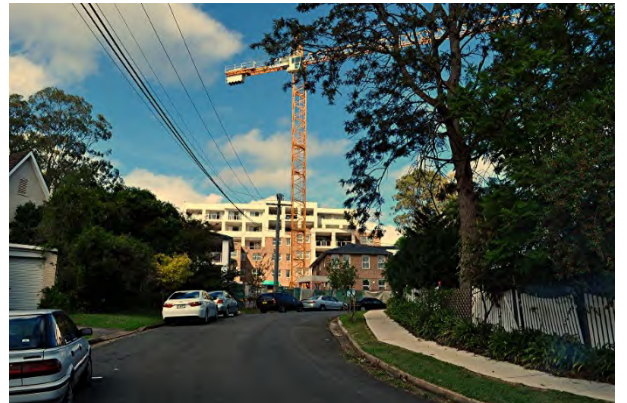
11. 9-13 Garthowen Crescent under construction.
