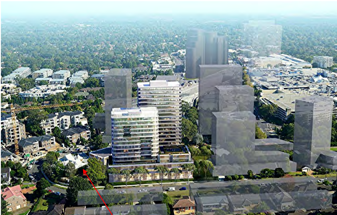
24. Aerial view from the north-east. “Garthowen”.
